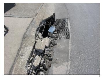
Fig. 15: Damaged curbs need maintenance.
