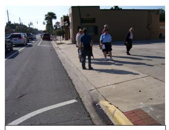
Fig. 18 Curb cuts are too wide and out of place.
