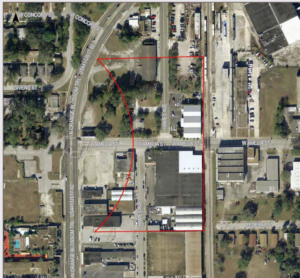
Aerial view of catalyst site and existing conditions
