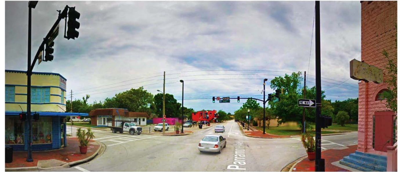
Exhibit III-14: Parramore Ave looking southbound: Existing conditions
