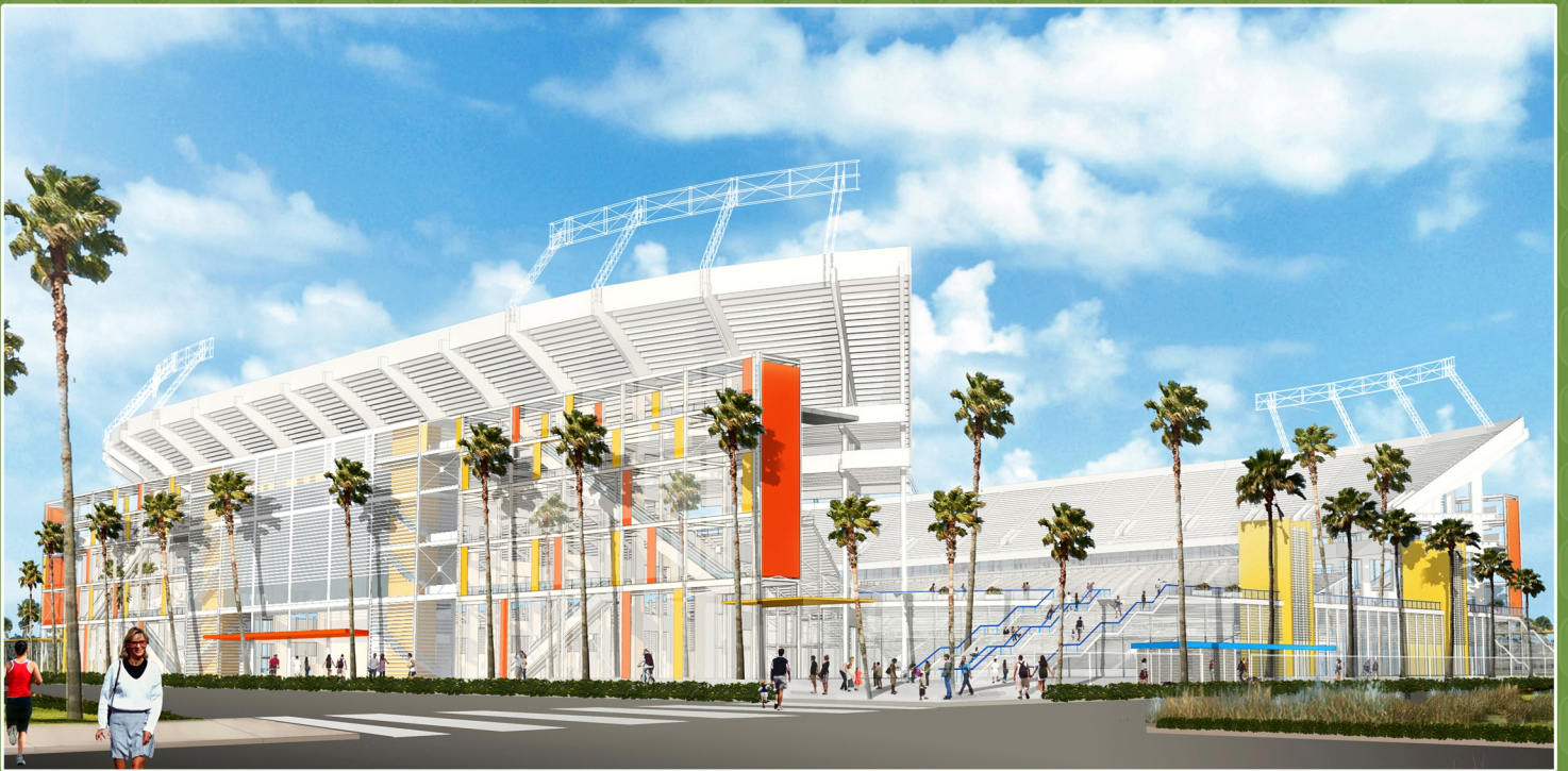
Florida Citrus Bowl Renovations
